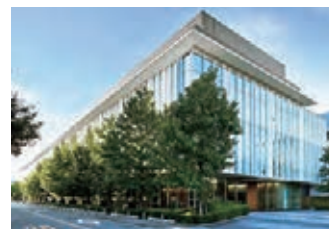
Manufacturing Technology Center (MTC)
