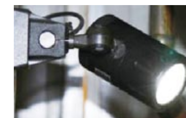
By changing lighting equipment to LED, Shimano Kunshan (China) reduced its monthly power consumption from 1625.4 kWh to 813.6 kWh.
