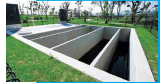
Oil-water separation reservoir: to prevent the inflow of untreated wastewater from the premises, the reservoir gathers and filters wastewater other than factory effluent.
