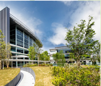
2020: Completed the head office R&D facility, “Technology Innovation Center”
